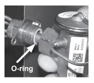
III-6. After ensuring that the Teflon O-ring seal is still in place inside the flowrator body, screw the female swivel nut onto the flowrator body.
